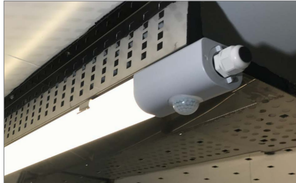
Lighting with motion sensor
