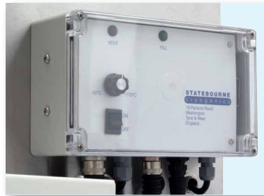
Hot gas by pass controls.
